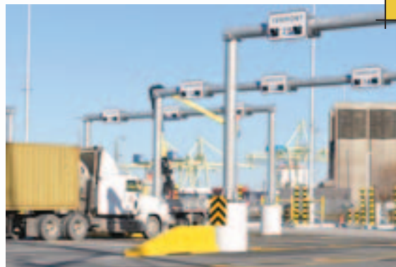
Port of Montréal Access and Security Upgrades, Montréal, QC
