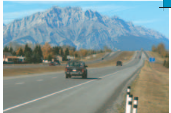
Trans-Canada Highway Improvements, Banff, AB
