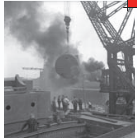
Marine crane loading boilers and engine assemblies at shipyard, 1943, Montréal, QC (photo courtesy of the National Film Board of Canada and Library and Archives Canada)
